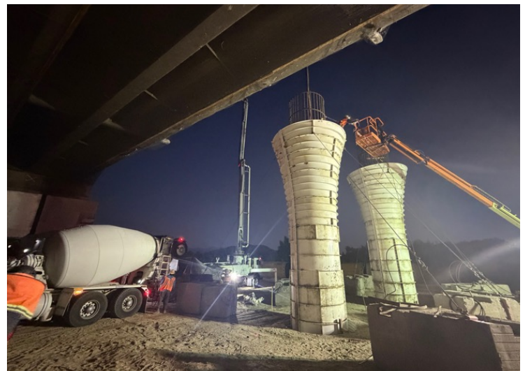
Concrete is placed for the northern bridge span support columns.
