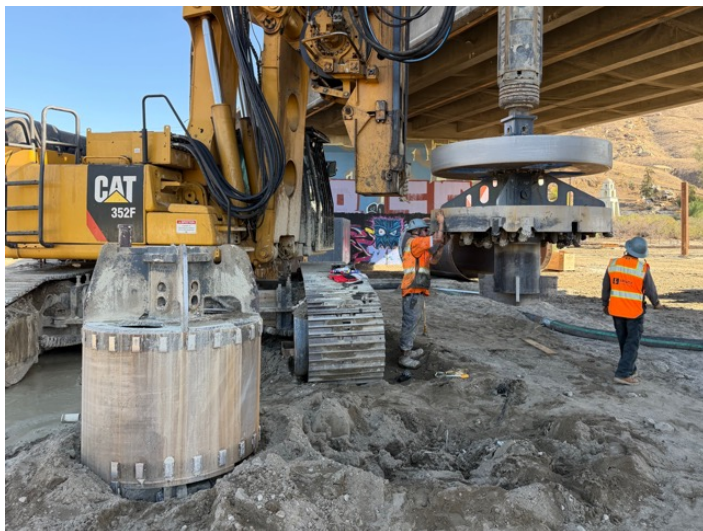
Crews perform drilling operations for the new bridge foundations.
